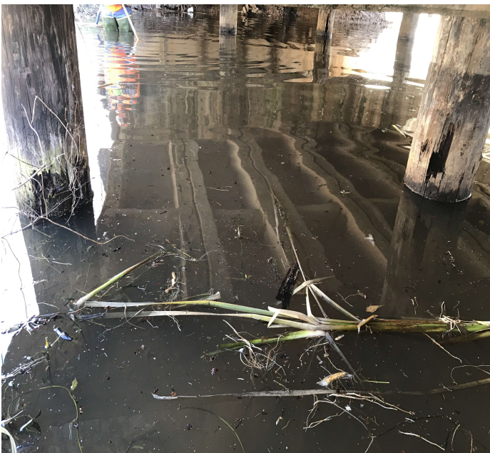
PHOTO 1 Description Bent 2 - Pile 1 & 2: Decay
